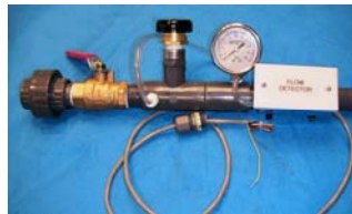
Flow Detector Assembly mounts in well line before it enters tank
